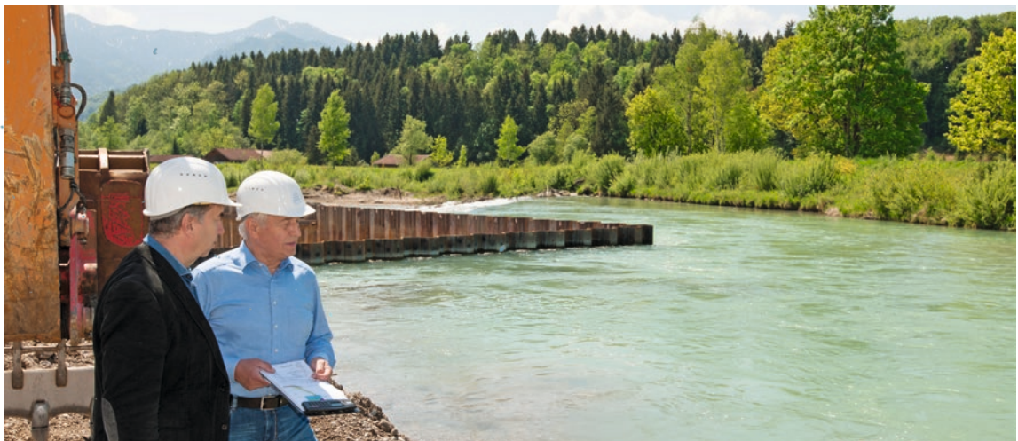
Engineers Albert Sepp (right) and Prof. Peter Rutschmann have developed the so-called “shaft power plant”. Construction of the demonstration plant at Grossweil could be an important step toward widespread use of this new hydroelectric power concept.
