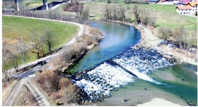
The first shaft power plant is to be built on the Bavarian river Loisach, using an existing weir.
