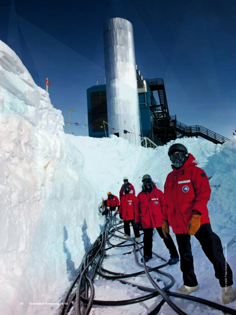
Pulling cables to connect the deployed sensors to the IceCube Lab in the detector's center. The 86 strings holding the sensors are distributed over an area of about one square kilometer. The lab houses data processing and storage and sends about 100 gigabytes of data by satellite every day.
